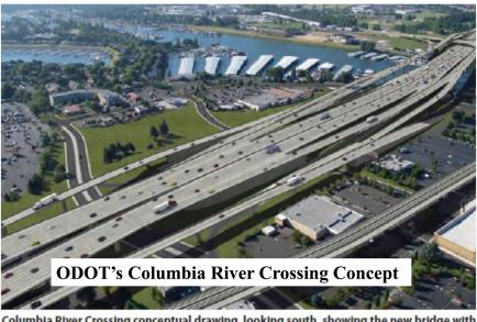
Columbia River Crossing conceptual drawing, looking south, showing the new bridge with light rail access along the west (lower right in drawing) side.
