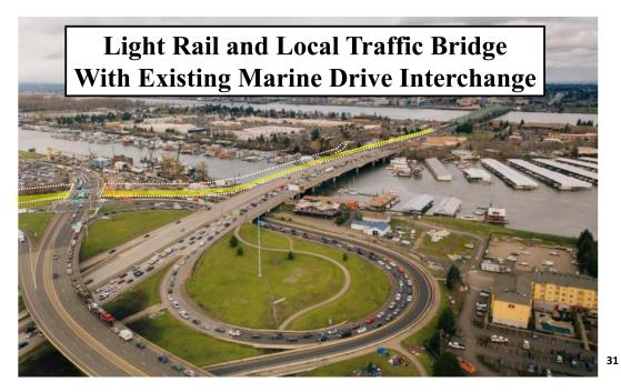
The CSA design of this interchange retains the existing infrastructure. The only difference is the extension of the MAX light-rail line and the addition of the new South Channel bridge, which is at the same level as the existing bridge.
