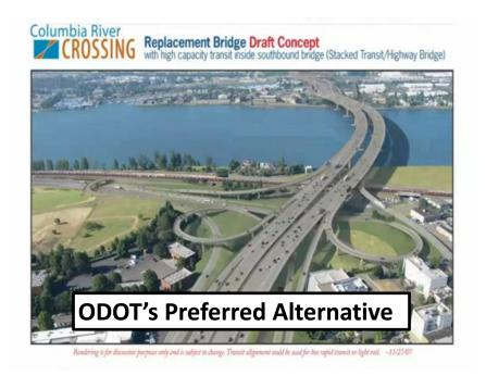
This is ODOT's illustration of the "Locally Preferred Alternative" looking south from Vancouver, showing the high-level approach to the bridge from Vancouver, and the steep, high-level on-ramps and off-ramps, towering above local buildings.
